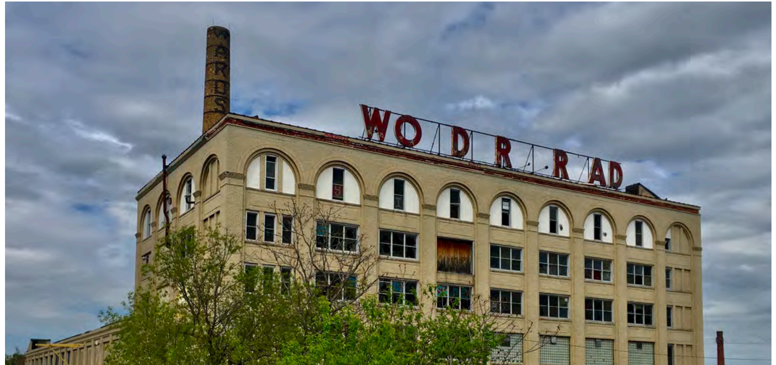
Former Wonderbread Factory. Photo: Google
